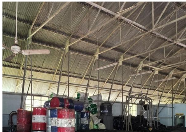
Figure 25: Improper storage of rubber waste within the processing area
