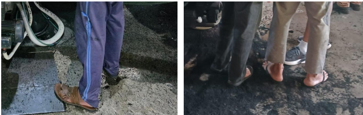
Figure 21: Operators working without safety shoes
